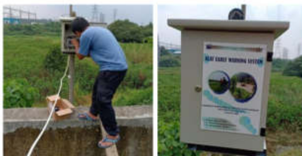
Gambar 3. Pemasangan alat early warning system (EWS)
