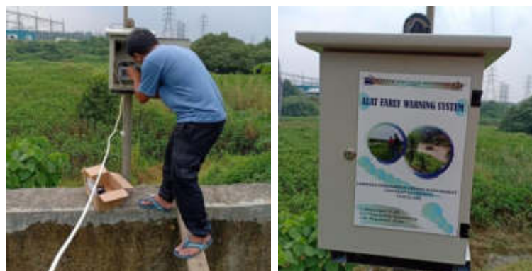
Gambar 3. Pemasangan alat early warning system (EWS)
