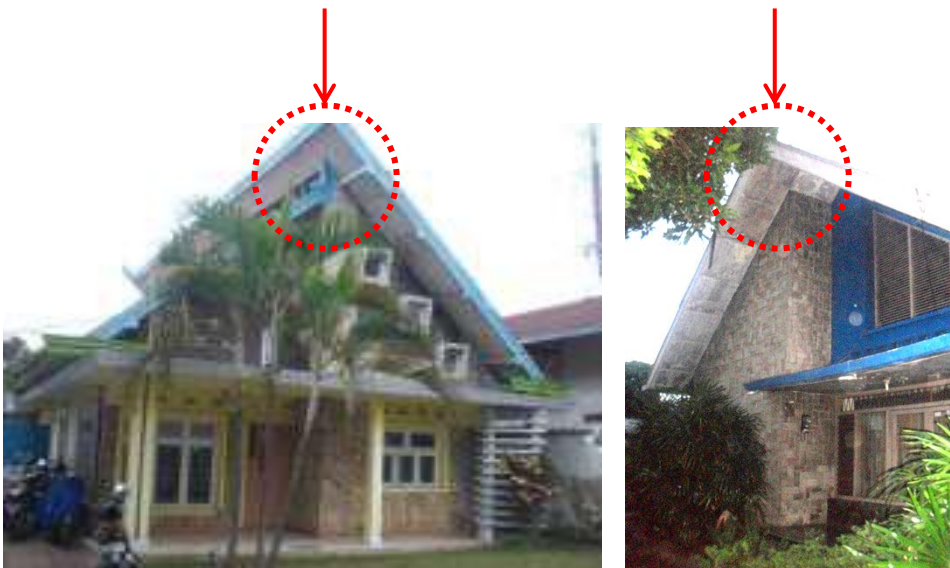
Picture 6. Difference of The Gable Roof in Malang Jengki House (left) and Pekalongan Jengki House (right) Source: Analysis from Susilo, et al, (2011) and Researcher, 2014
