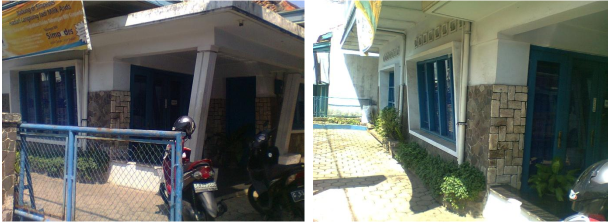
Picture 4. Other Variant of Jengki House in Pekalongan Source: Researcher's Field Survey, 2014
