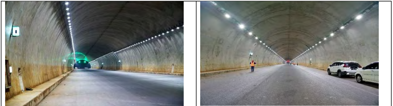
Fig. 2 Inside Cisumdawu Tunnel
